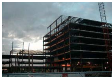
5 Figure 3. VEC Steel Erection
